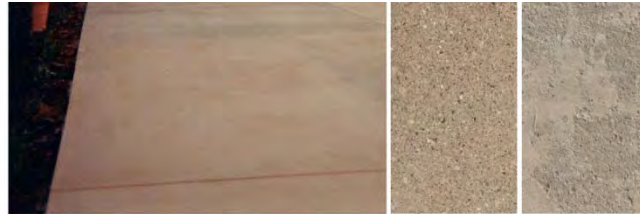
Rustic concrete finishes (e.g., tan-colored concrete with light sandblasting) such as those pictured above would help maintain Boonville's rural character.
