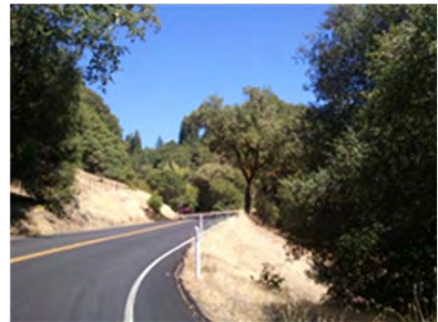
SR 128 becomes winding and steep between Boonville and the Sonoma County line (Segment 5).
