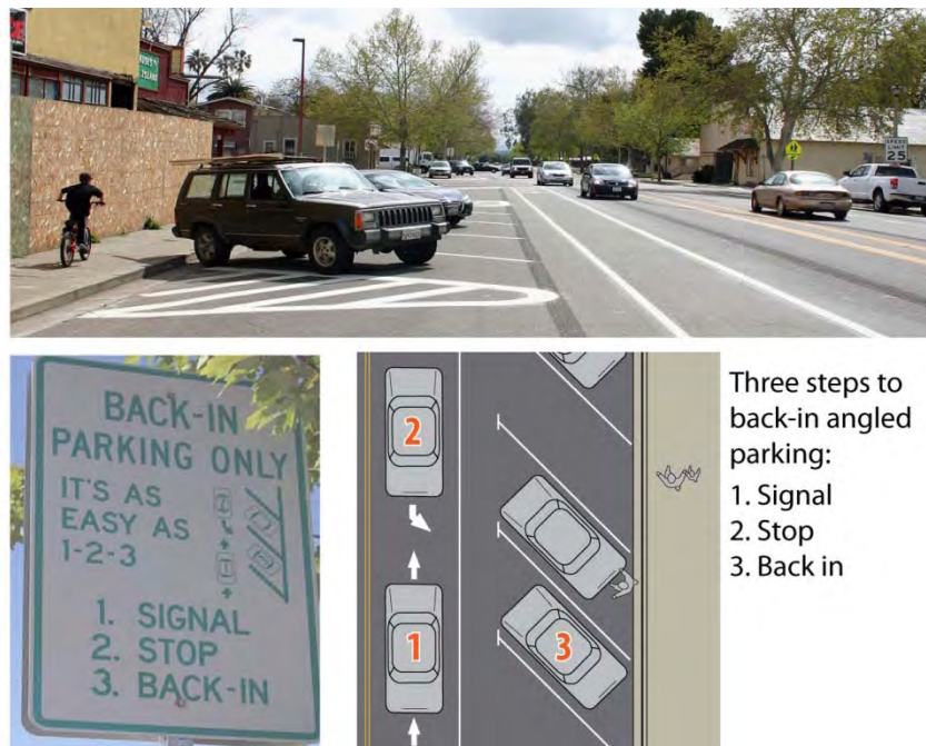
Figure 7-18: Back-In Angled Parking Allows Drivers a Clear View of Oncoming Vehicles and Bicyclists
