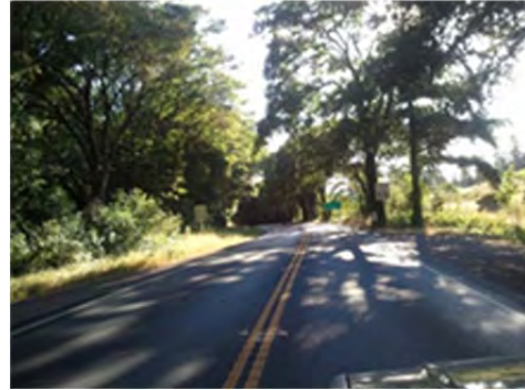
SR 128 between Philo and Navarro (Segment 2).
