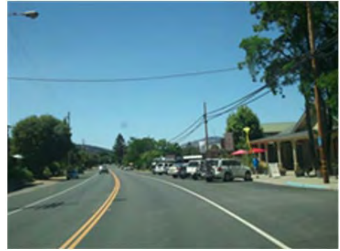
SR 128 through downtown Boonville (Segment 4).
