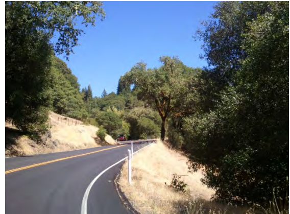
SR 128 is a primary route between U.S. 101 and the central Mendocino Coast. It also serves as the "Main Street" and is virtually the only route for travel between Anderson Valley's rural communities of Navarro, Philo, Boonville, and Yorkville.
