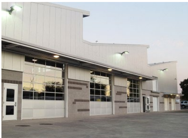
MTA Maintenance Facility. Source: LSC Transportation Consultants, Inc.
