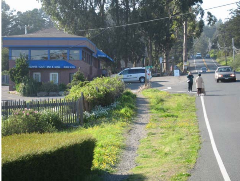
Foot path warn into soft shoulder southwest of Ocean Drive
