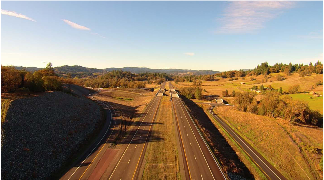
Willits Bypass northbound: Southern Interchange
