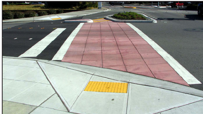
The photo to the right illustrates a low speed entry ramp accentuated by a raised crossing to assure low speeds.
