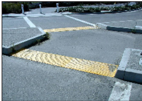
Tactile edges allow the vision-impaired to sense the edge of the "safe zone" for pedestrians and know they are crossing traffic.
