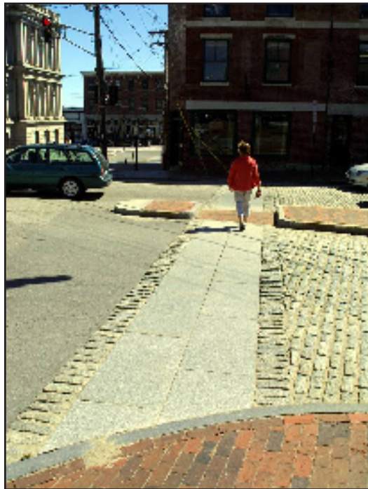
ADA requirements were often originally met in haste without proper alignment of paths. Many municipalities are now correcting these placements.
