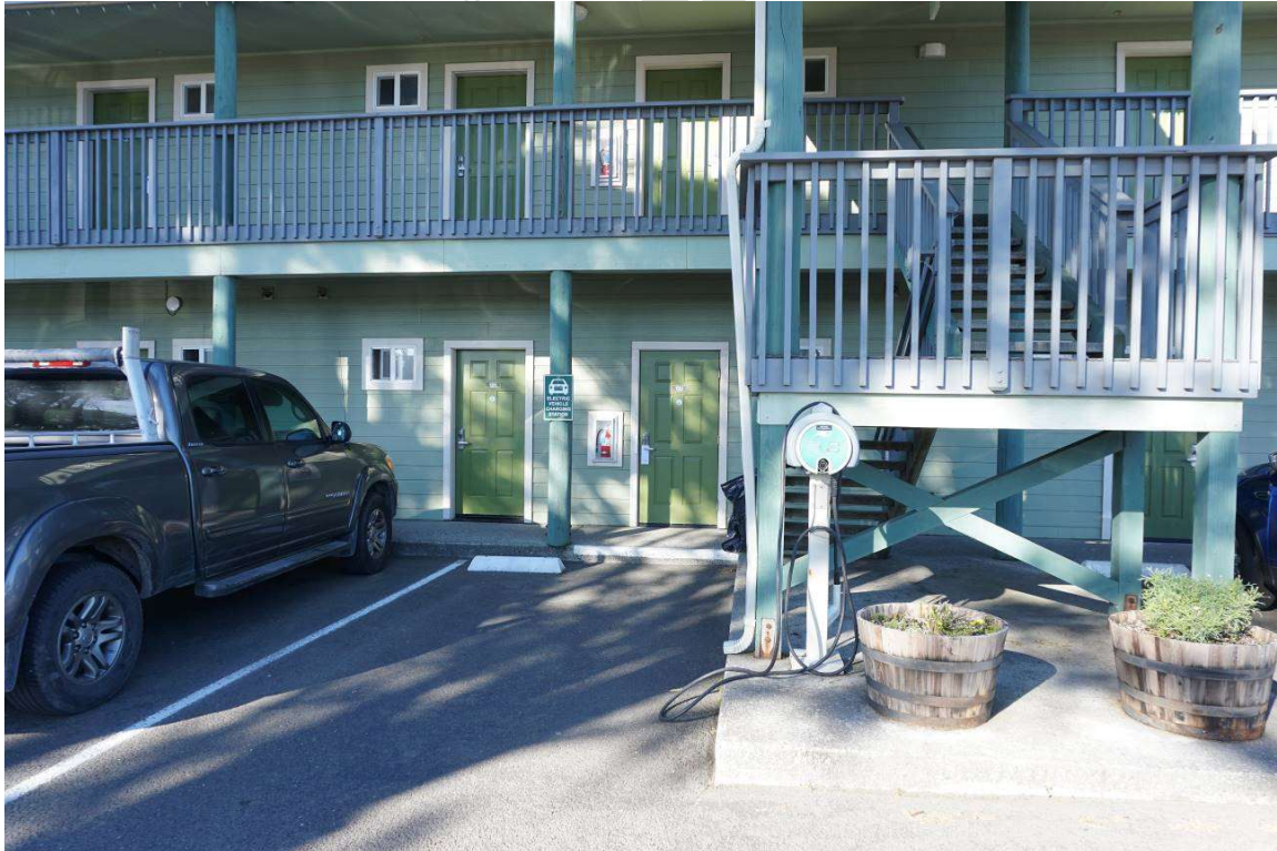
Plate 4 Level 2 charger at a hotel in Fort Bragg
