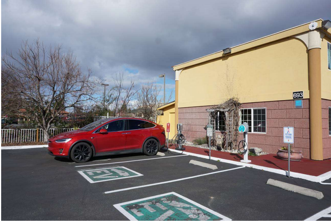
Plate 13 Level 2 chargers at Super 8 Motel in Ukiah
