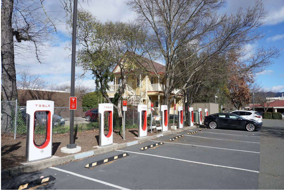
Plate 2 Tesla Superchargers in a City Ukiah parking lot
