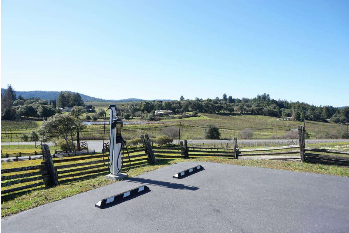
Plate 9 Level 2 charger at Handley Cellars in Philo
