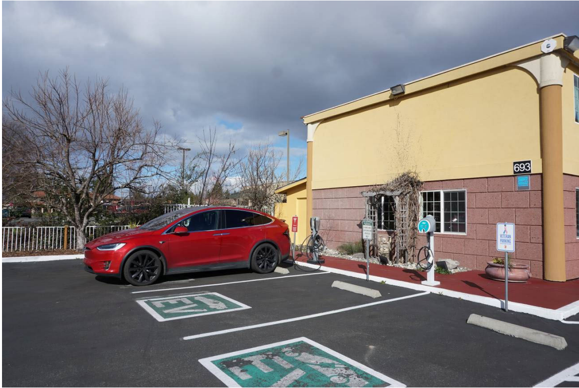
Plate 15 Level 2 chargers at Super 8 Motel in Ukiah
