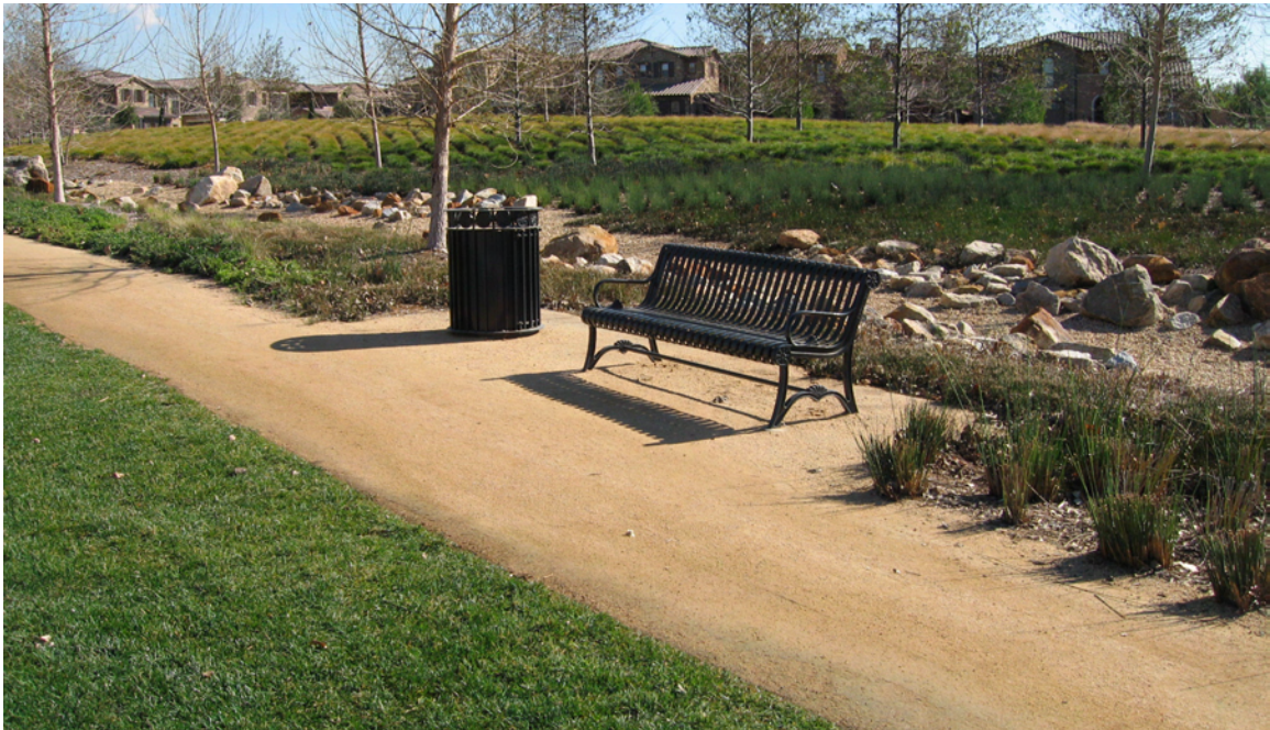
Stabilized Compacted Material
