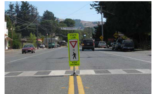
Pedestrian signage in advance of a crosswalk
