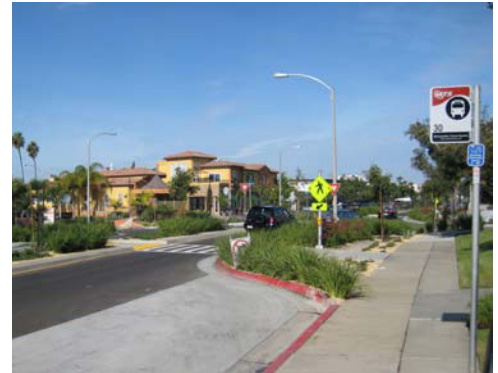
Bulbout with high visibility crosswalk
