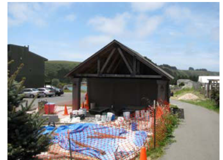
Current construction of the Centennial Plaza Memorial Garden
