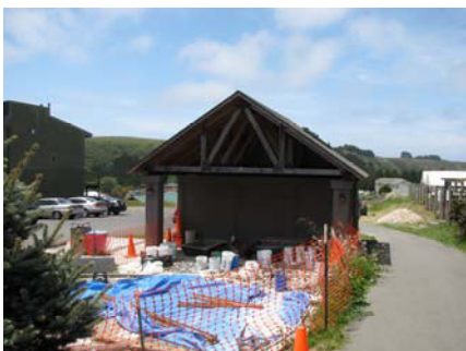
Centennial Plaza Memorial Garden under construction
