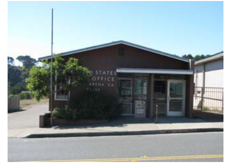
Existing post office
