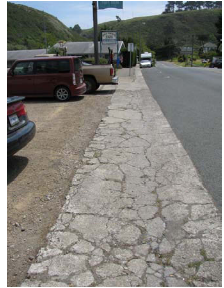
Existing sidewalk conditions
