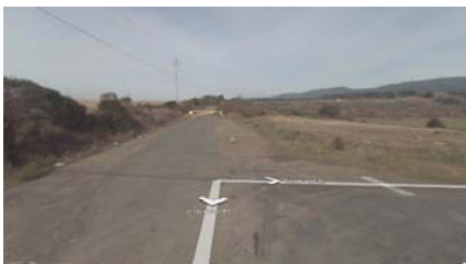
Site of bridge removal on Windy Hollow Road (source: maps.google.com)
