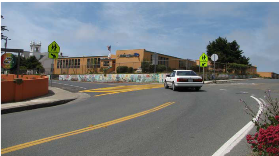
The Main Street/Lake Street/School Street intersection has limited sight distance for pedestrians and vehicles
