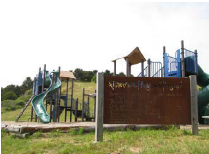
Recently constructed Fisherman's Playground Project
