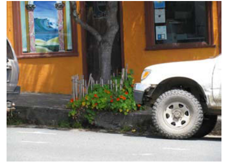
High curbs in downtown Point Arena are difficult to navigate
