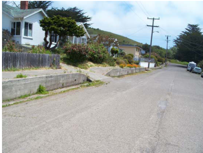
Sidewalks on Mill Street
