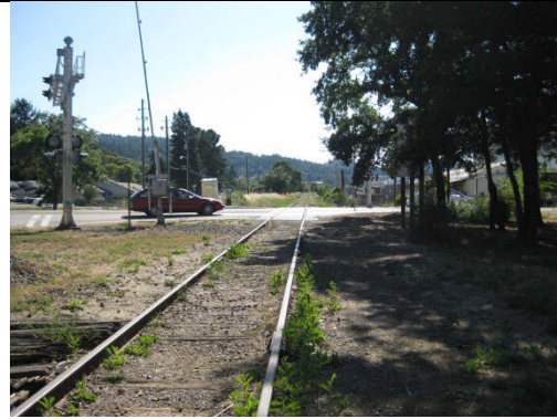
NWP Corridor/Highway 101 intersection (facing west)
