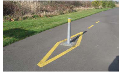
A retroreflective pavement striping pattern brings attention to this bollard
