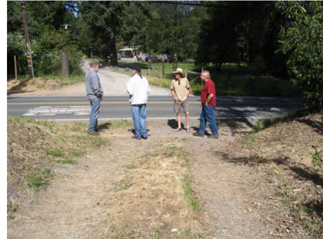
Segment #3 – There are two driveways where resolving walkway (running left-to-right across the driveway) slopes approaching the driveway will require re-grading of the walkway approaches to the driveways.
