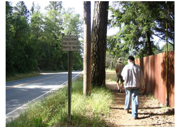
Segment #4 – This photo is taken looking south on the west side of Branscomb Road toward the crosswalk that forms the southern limit of this reach. While there are obstacles, including fences and trees, there is sufficient space to add a four to six-foot walkway.
