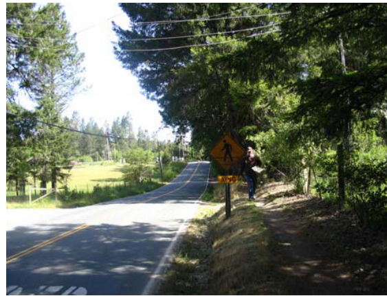
Segment #3 – This photo is taken looking north on the east side of Branscomb Road toward the crosswalk that forms the northern limit of this reach. In several places, the walkway will be above roadway and separated by a natural drainage swale. One reason for selecting a crushed rock trail surface is to simplify maintenance in the event that the slope sloughs off.
