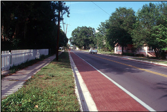
Colored shoulders on a State Highway in Florida (source: pedbikeimages.org / Dan Burden)
