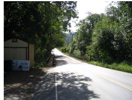
Segment #5 – This photo is taken looking west on the north side of Branscomb Road with the Ten Mile Creek walkway just beyond the pedestrians. There is little separation between the walkway and high speed vehicles.
