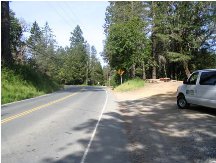
Segment #4 – This photo is taken looking west on the north side of Branscomb Road at the Bauer Road intersection and curve. The trail would be located in the shoulder area. It would be desirable to re-grade the outside edge of the curve to add super-elevation.
