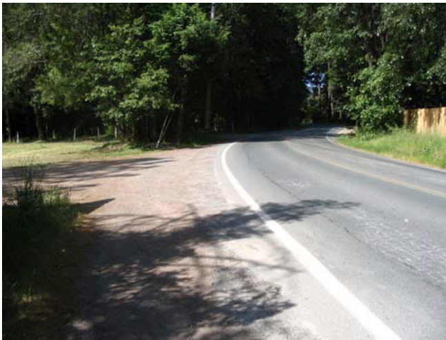
Segment #2 - Branscomb Road looking west at and beyond the Laytonville Cemetery driveway. The current walkway transitions from the south to the north side of the street, but with proposed improvements would continue on the south side behind and among the trees on the left-hand side of this photo.
