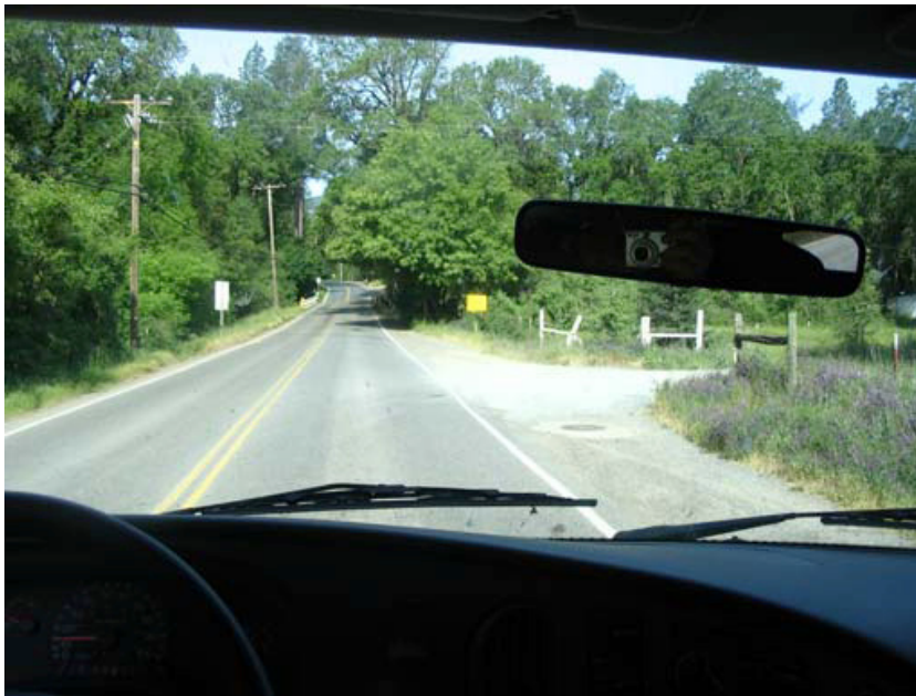
Segment #6 – This photo is taken looking west on the north side of Branscomb Road with the Ten Mile Creek walkway in the distance. There is sufficient shoulder width to accommodate a walkway located adjacent to the roadway.
