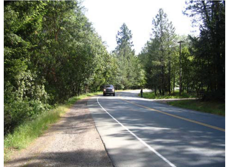
Segment #4 – This photo is taken looking north on the west side of Branscomb Road at the curve after Bauer Road is behind. The trail would be located in the shoulder area. It would be desirable to re-grade the outside edge of the curve to add super-elevation.
