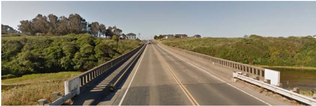
Existing Bridge - Looking South
