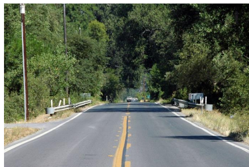
Natural features, such as Mill Creek, can present challenges for trail planning and implementation.
