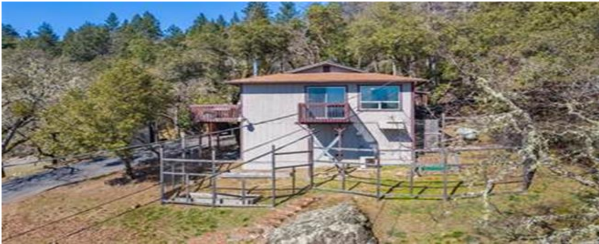
Typical residence and fuel type in Fire Model area #2
